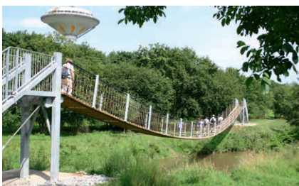
Wooden walkway bridge, Length 54 m
