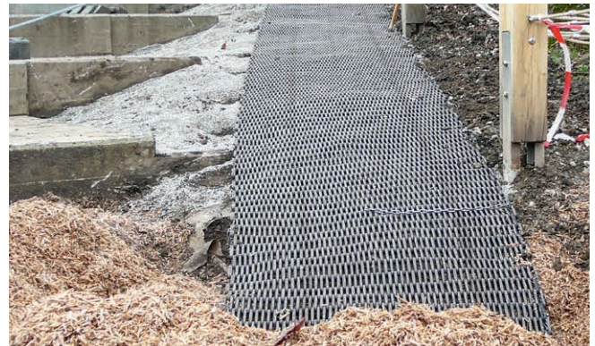
Mat directly after placing
