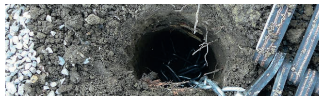
Small hole in ground for anchor chains + point foundation (ca. Ø 5.00 cm)
