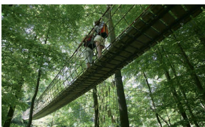
Wooden walkway bridge, Length 40 m
