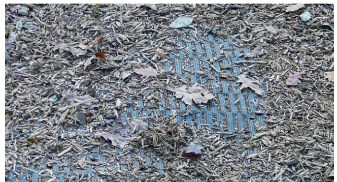
Lawn protection mats after installation (laid open for photo)
